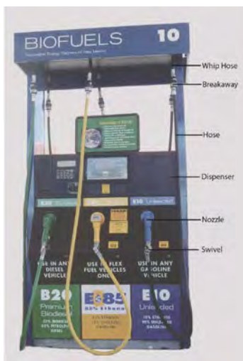
Figure 5. Aboveground equipment
